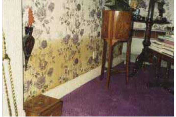
The 2007 edition of Digest 245 says this is a wall with rising damp (left image) but BR466 Understanding dampness says this is not a case of rising damp (right image) but is due to animal urine
