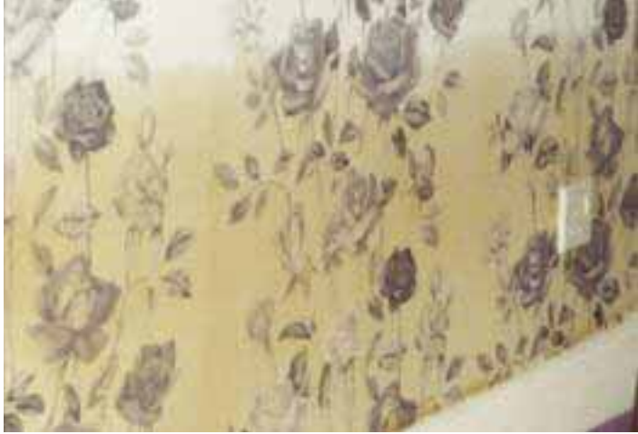
The 2007 edition of Digest 245 says this is a wall with rising damp (left image) but BR466 Understanding dampness says this is not a case of rising damp (right image) but is due to animal urine
